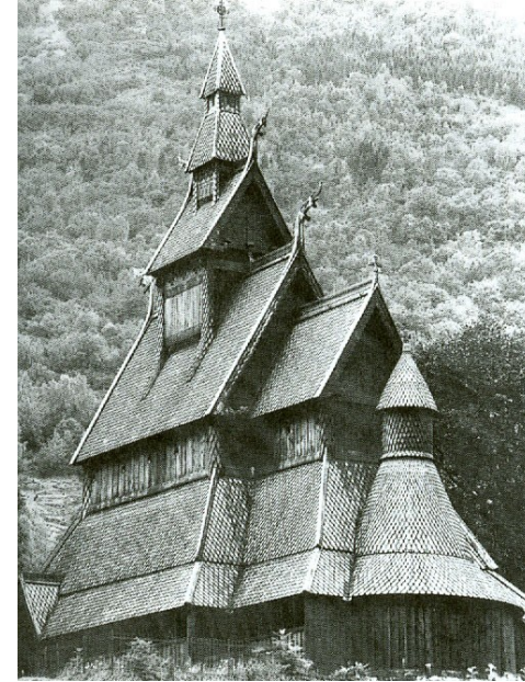
Roofs of a norwegian stave church
